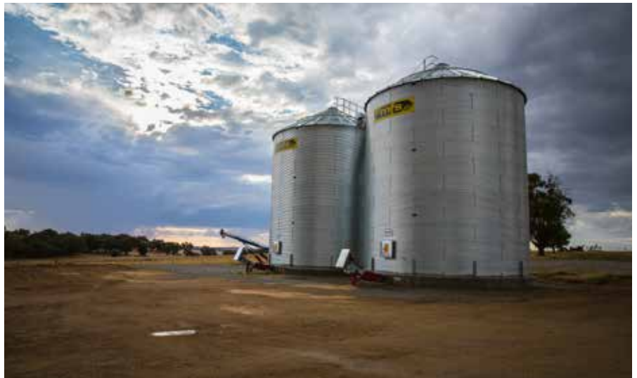
Allied Grain Systems sits at the very top of their field – they are one of the top companies in Australia making grain silos and grain handling equipment.
